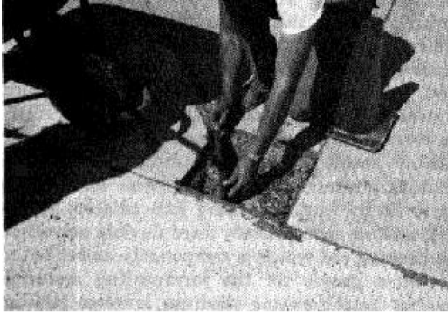
Figure 3. Placement of joint filler sheet to maintain active crack through area to be patched.
